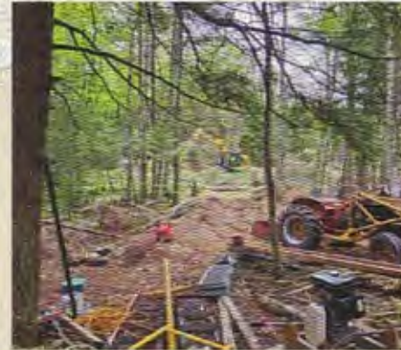
Clearing, grubbing, and moving the old bridge
